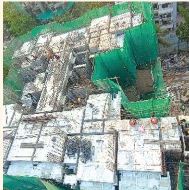
Wing - B : Top View 8 th Slab Reinforcement Work in Progress
