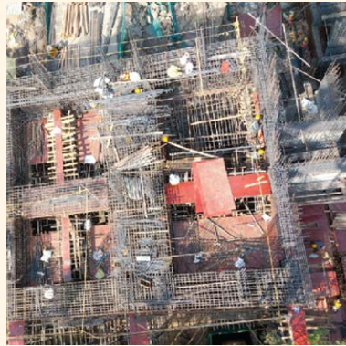
Wing G & F 2 nd Podium Slab Work in Progress
