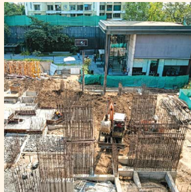
Wing - A & B: Plinth and Column Work in Progress
