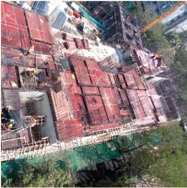
Wing A, B & C 6 th Floor Slab Work in Progress
